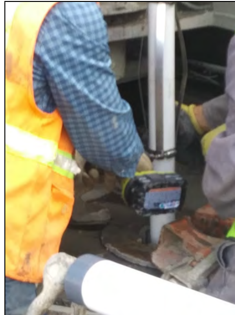
Centralizers are installed every 10 feet within the screened section, and every 80 feet along the rest of the casing.
