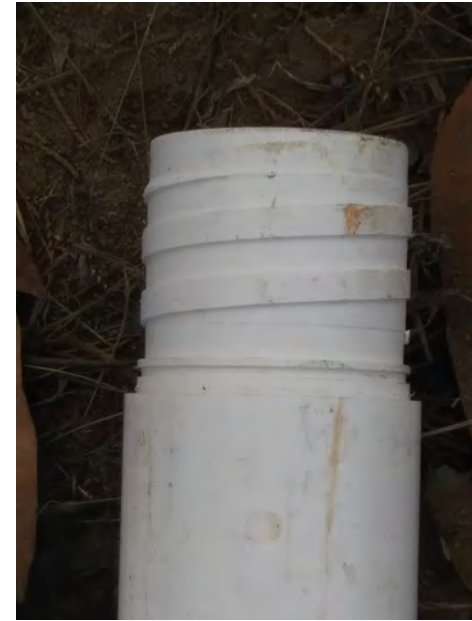
Installing the 2" Schedule 80 PVC Casing. The joints are flush threaded.
